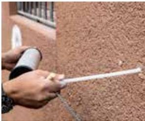
Clean hole with a blow pump (>2x) and a brush (>2x).
