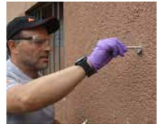
Insert the anchor with a rotary motion.
