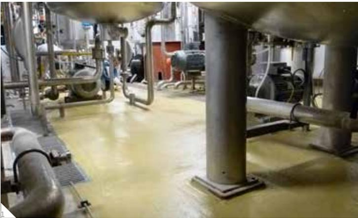
**1.** Chemical processing plant. The electric conductive Sikafloor® PurCem® HS-25 ECF withstands the spillage and leakages from the process and controls the static electricity discharge.
