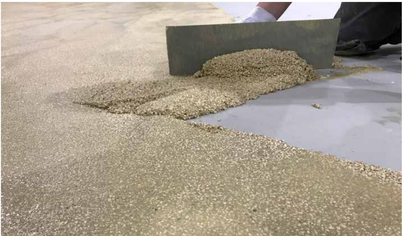
Sikafloor® PurCem® HM-20 HSR is a textured trowel-grade system with high slip resistance. Typical application is done with a trowel or “screed box.”
