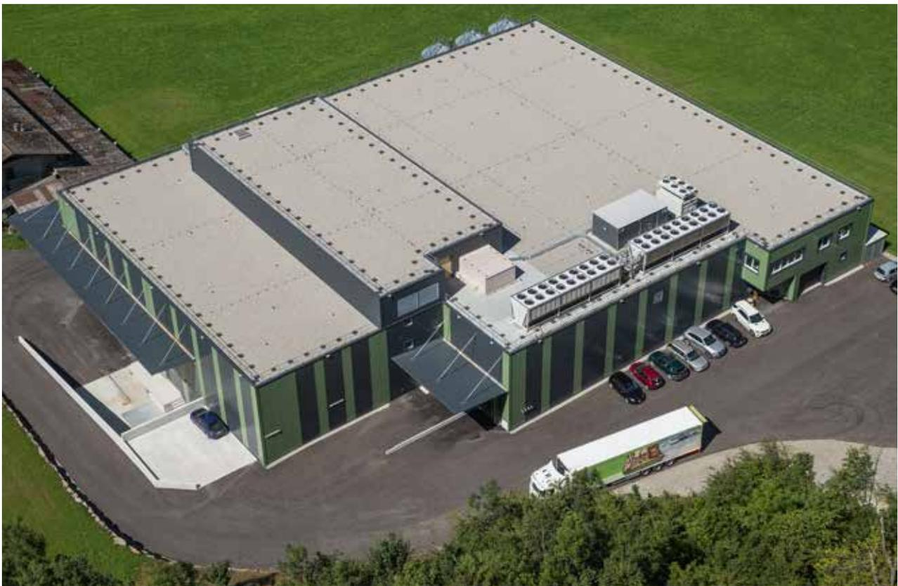
To resist wind uplift the membranes are either mechanically fastened or fully adhered to the roofing structure. Mechanical fastening offers a fast and cost efficient application whereas an adhered solution meets high aesthetic requirements and freedom to design complex roof shapes.
