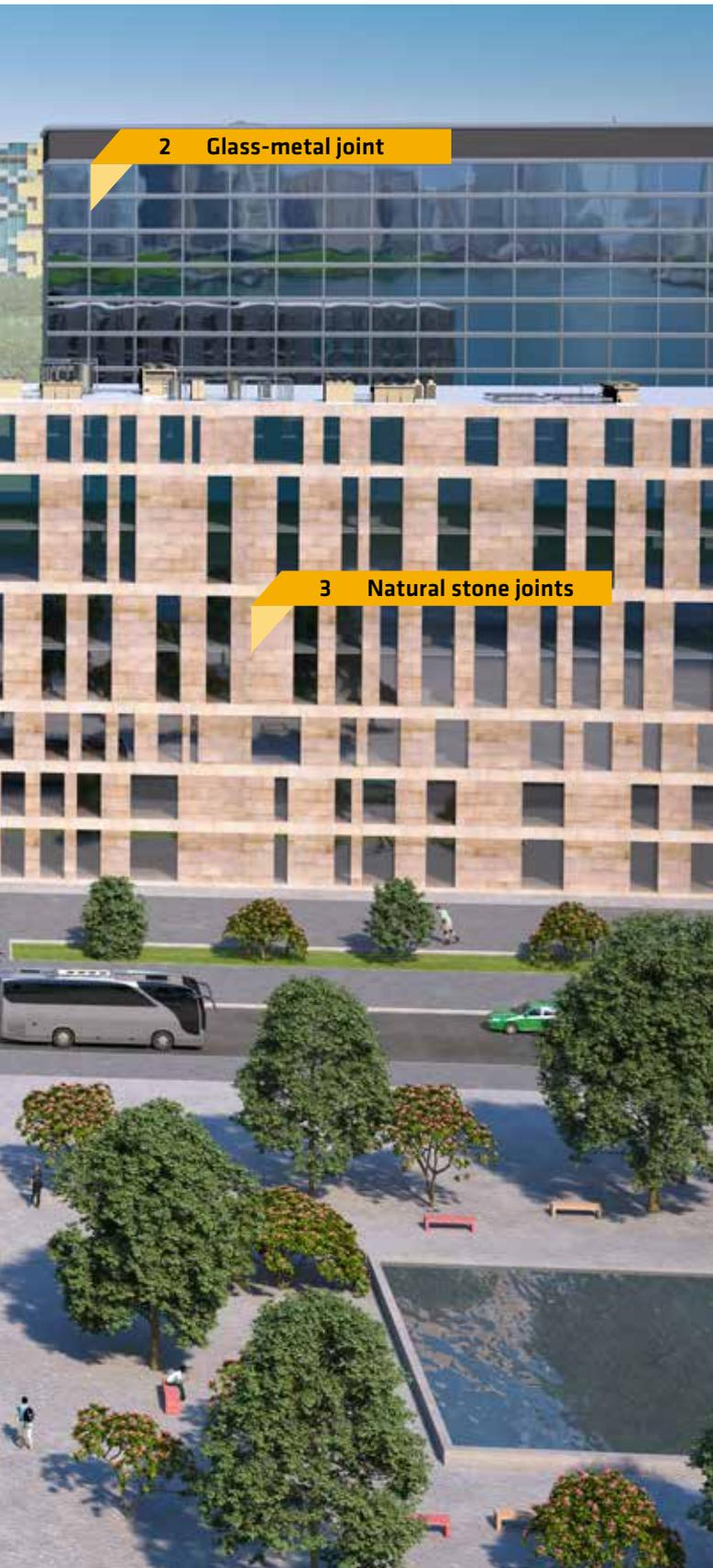
ALL THE DIFFERENT ELEMENTS, MATERIALS AND TRADES MEET AT THE JOINTS – THINK ABOUT JOINT SEALING SOLUTIONS EARLY FOR A WATERTIGHT BUILDING ENVELOPE!
