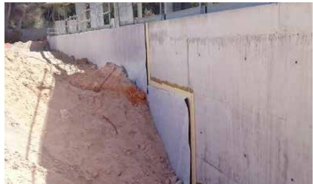
For open excavations: The protection of the SikaProof® membrane is mandatory, especially regarding the backfilling.
