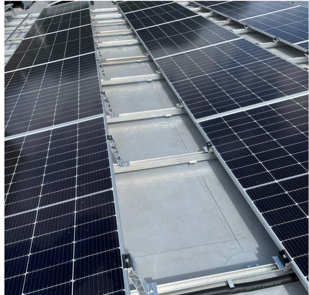
Due to the M12 inside thread, it is easy to assemble a broad range of solar construction onto the SikaRoof® Anchor System.
