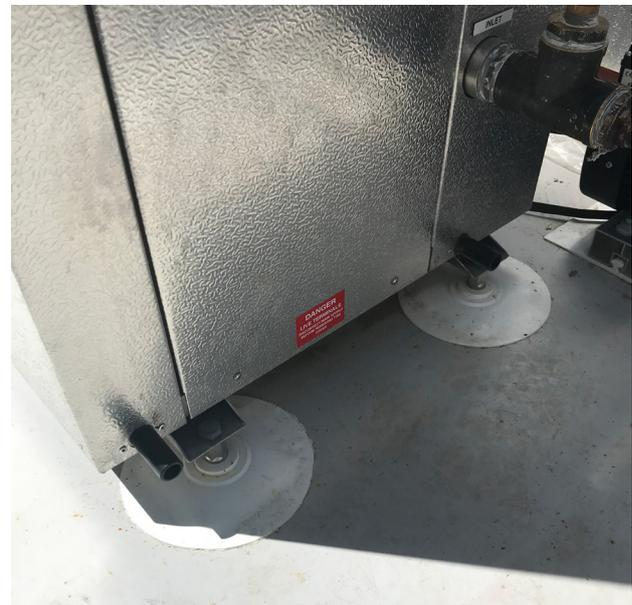
Versatile installation of various appliances / equipment onto the SikaRoof® Anchor System.
