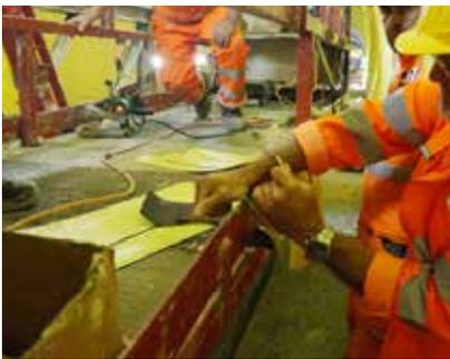
Peel tests have to be performed on separate membrane samples at the beginning of each membrane application to set the machine parameters, as well as at regular intervals during the application to adjust the welding setup according to the changing climatic conditions.
