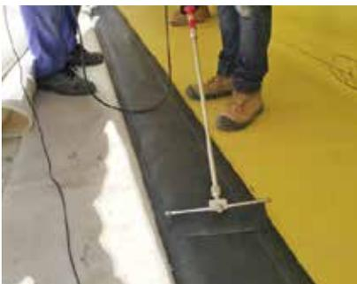
Area defect testing with an electrical copper wire brush holiday test. Electrical sparks signalizes capilarities in seams. Any defects in the membrane or at seam edges can be detected, if an electrical conductor is placed underneath.
