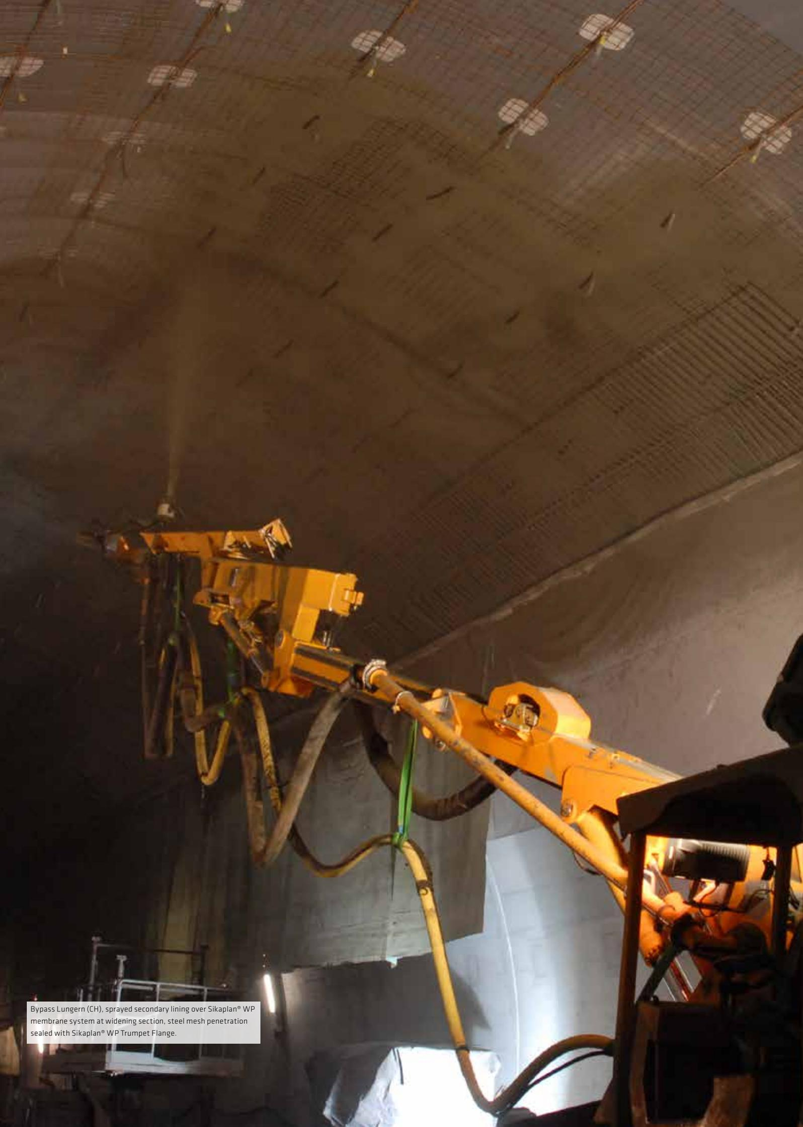
Bypass Lungern (CH), sprayed secondary lining over Sikaplan® WP membrane system at widening section, steel mesh penetration sealed with Sikaplan® WP Trumpet Flange.
