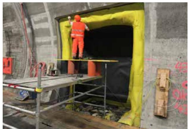
Waterproofing of the excavated tunnel niche using Sikaplan® membrane, directly connected to the existing PVC membrane.
