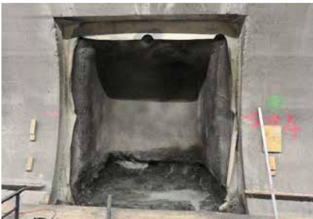
Excavated niche during maintenance works allows accessibility to 44 years old exposed Sika membrane for durability testings.
